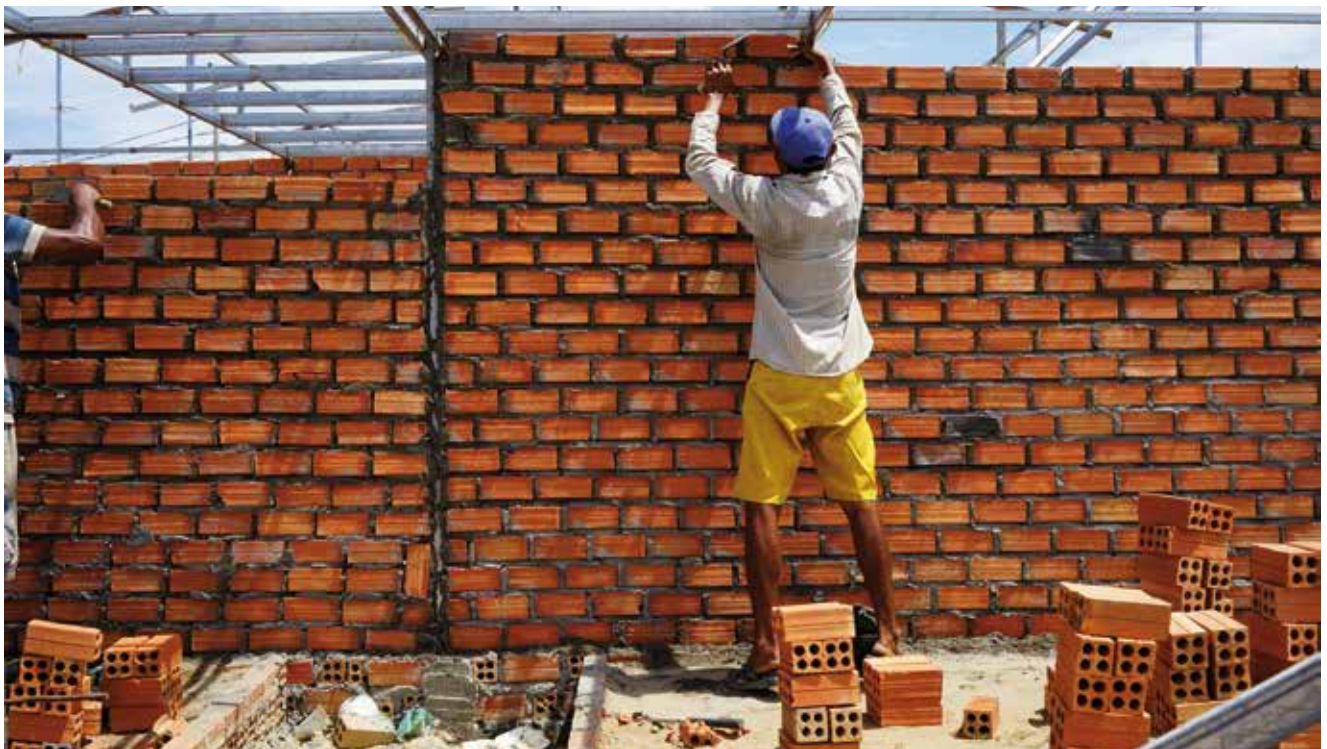
Figure 5: Burnt clay bricks are still the dominant construction material in Cambodia
