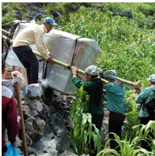
Figure 3: Transportation of a switchboard (207 kg)
