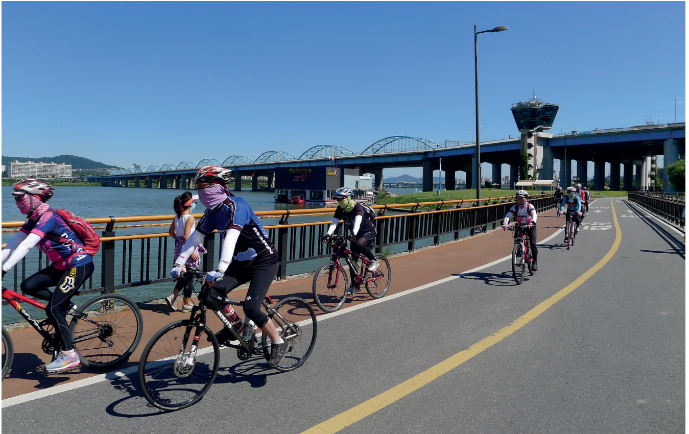
Figure 2: Bicycle Lanes along the Hangang River.
