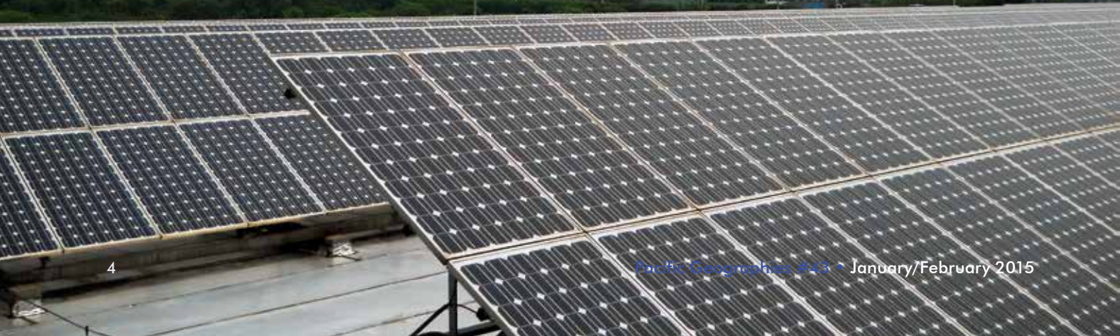
Figure 1: PV Panels in North China
