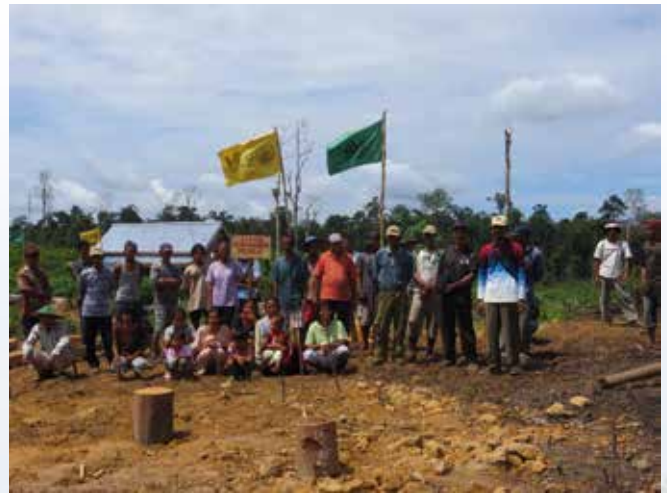
Picture 4: SPI Members at a Mosque construction site within Hutan Harapan
